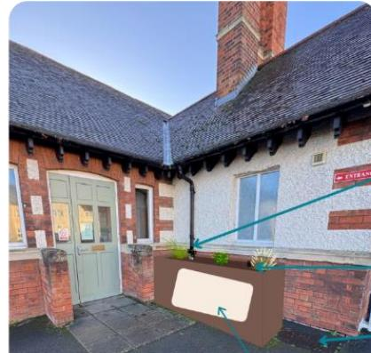
Downpipe/drain pipe cut and diverted into rain garden
