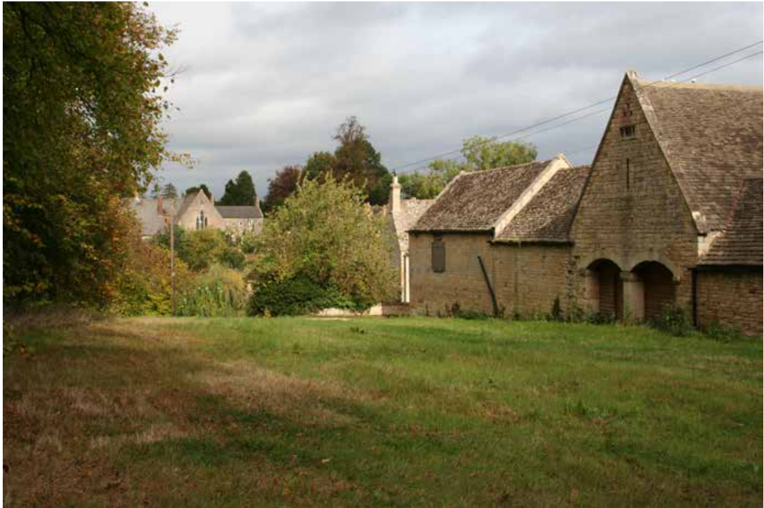
Photograph 5: A view along the valued façade of Almsbury Farm along Vineyard Street
